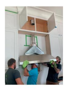
Whether venting through the wall or cabinetry or ceiling, make sure the hole for the ducting is cut before attempting to install the range hood. Test fit the ducting being used for fit through the hole. It should not be tight around the ducting.
