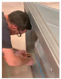
Additional ducting should be added to the liner (or transition unit, if applicable). If the liner is being vented into the wall, this will include an elbow and at least enough horizontal ducting to exit through the wall. If the liner is being vented through the ceiling, make sure there is enough vertical ducting to reach the upper level so the remaining ducting can be sealed and continued.
